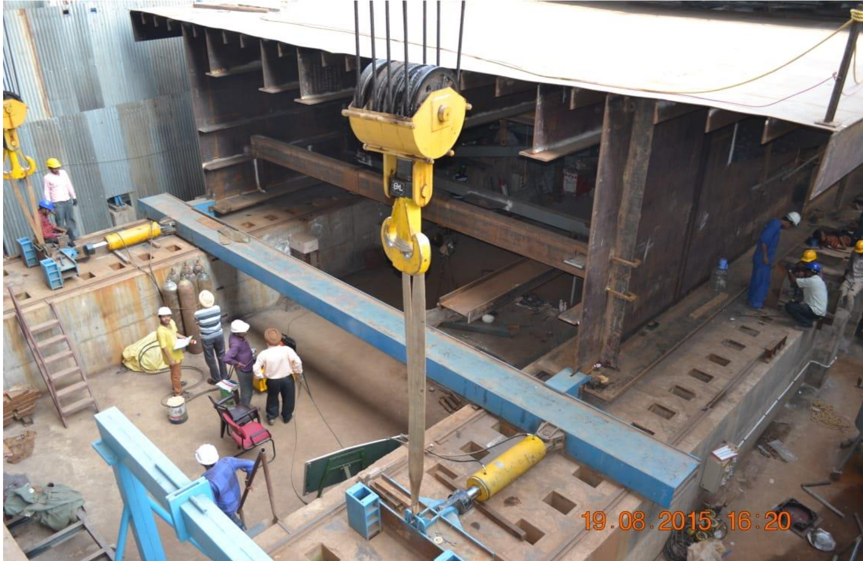
Pushing of Segment Arrangement @ S180 Abutment
