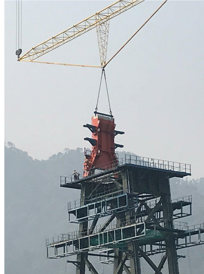
Erection of Temporary tower on Pier in progress
