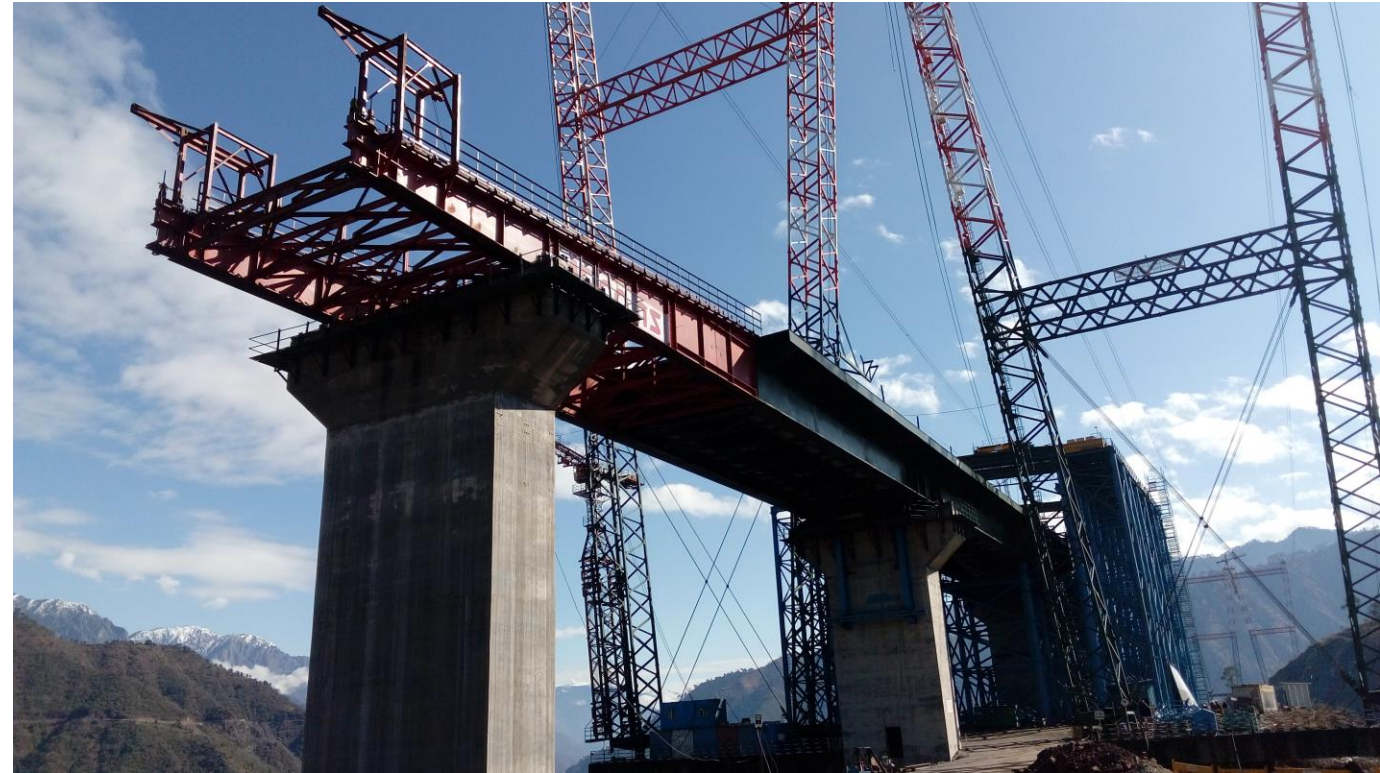
Incremental Launching of Viaduct Span in Progress
