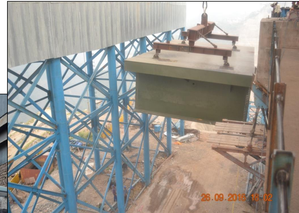
Lifting of Segment on Platform
