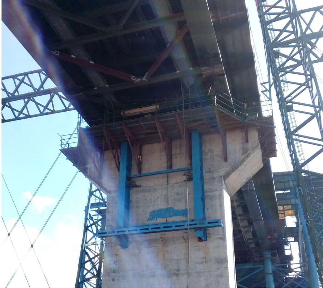
Puling Arrangement @S90 Supporting frame & Strand Jacks added on Pier S90
