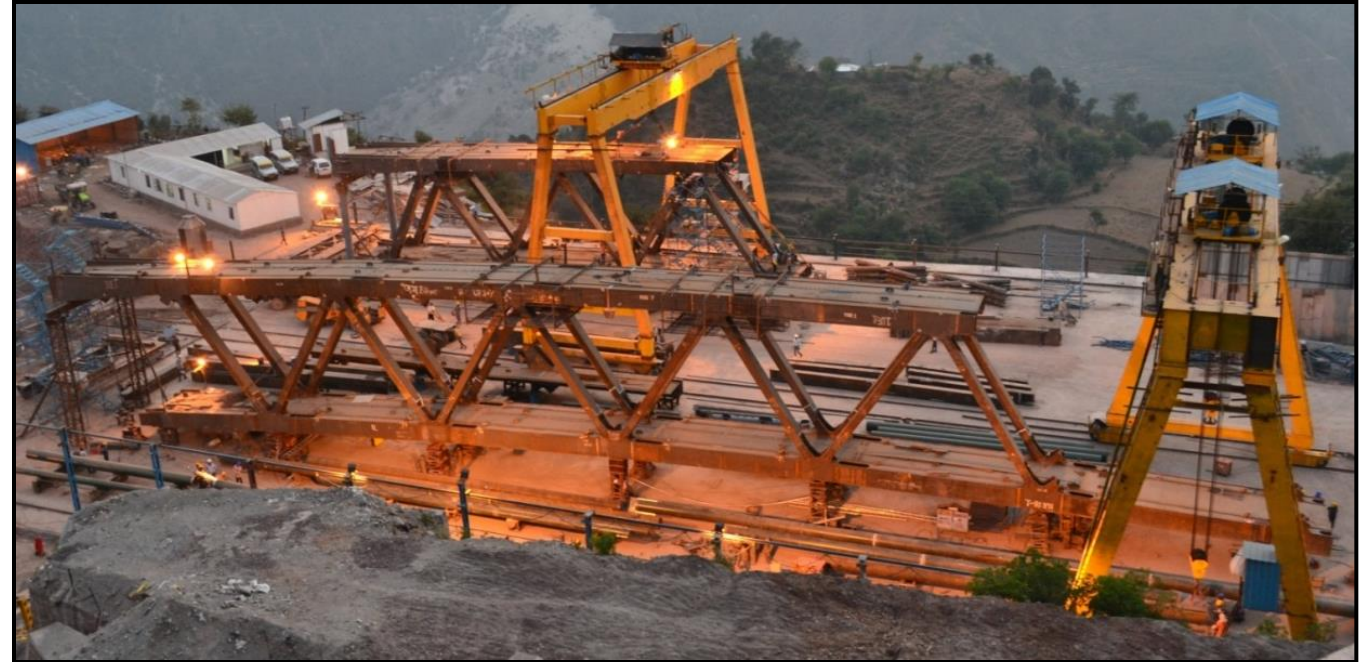
Full scale trial assembly of Arch
