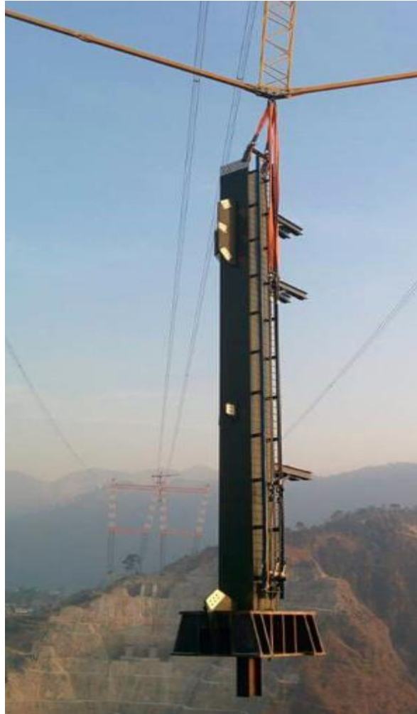
Erection of Pier Base Segment
